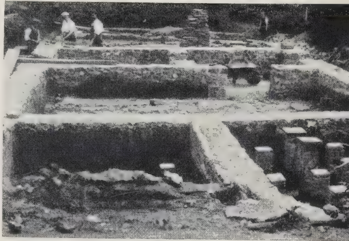
Excavating Newport Villa—hypocaust at lower right
